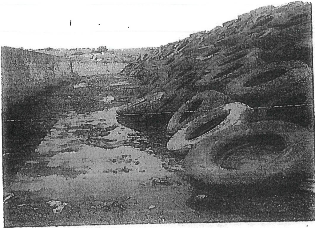
Photo 1: Silage pit made on gravel base with no silage effluent collection channels in place.
